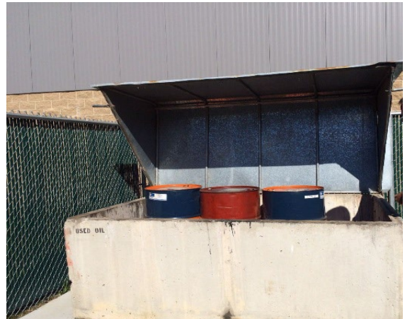
Proper outdoor storage of used oil containers – containers are protected from precipitation and are stored on an impervious surface.
