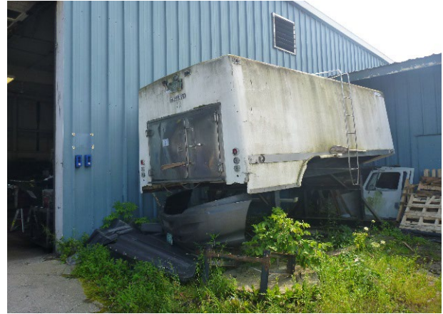
Improper secondary containment for aboveground storage of used oil outdoors - single-walled, unlabeled tank containing used oil.
